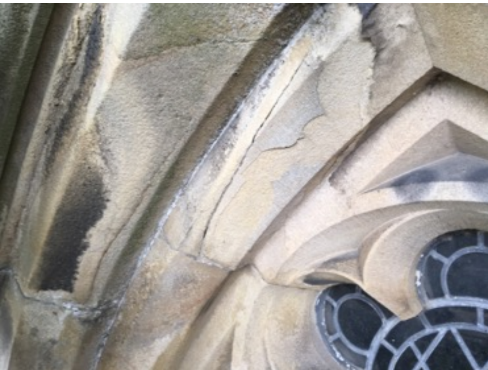
Cracked inner moulding to main west window upper section below pointed arch.
