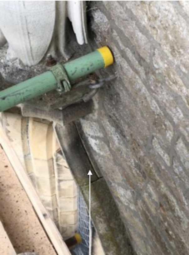
Cracked hood moulding to the main west window
