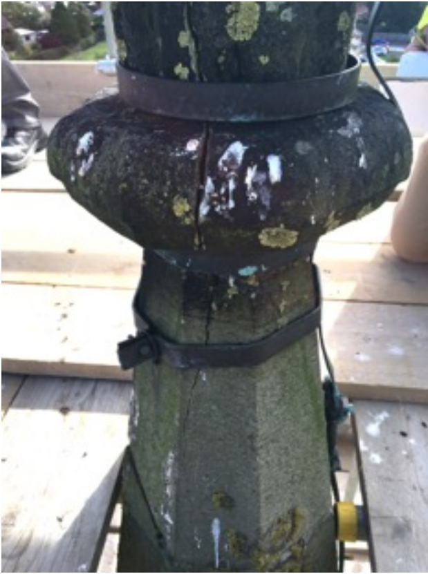
Cracked pinnacle stones
