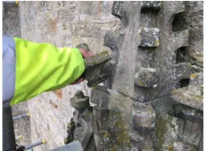
Loose cross pieces to west pinnacle above statue
