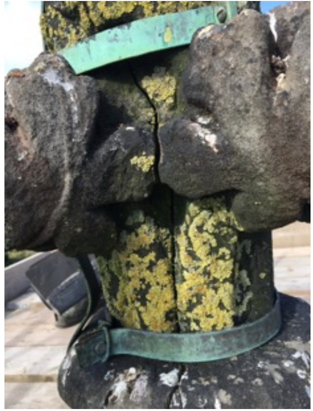
Cracked pinnacle stones
