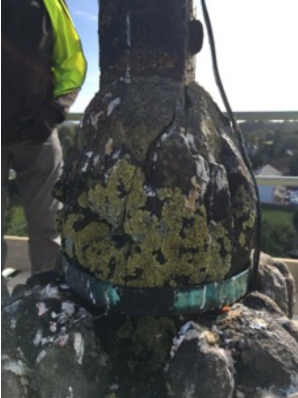
Cracked pinnacle summit stone with concrete fill to ferrous block.
