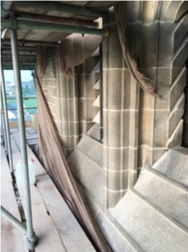
Belfry opening pointing and new louvres
