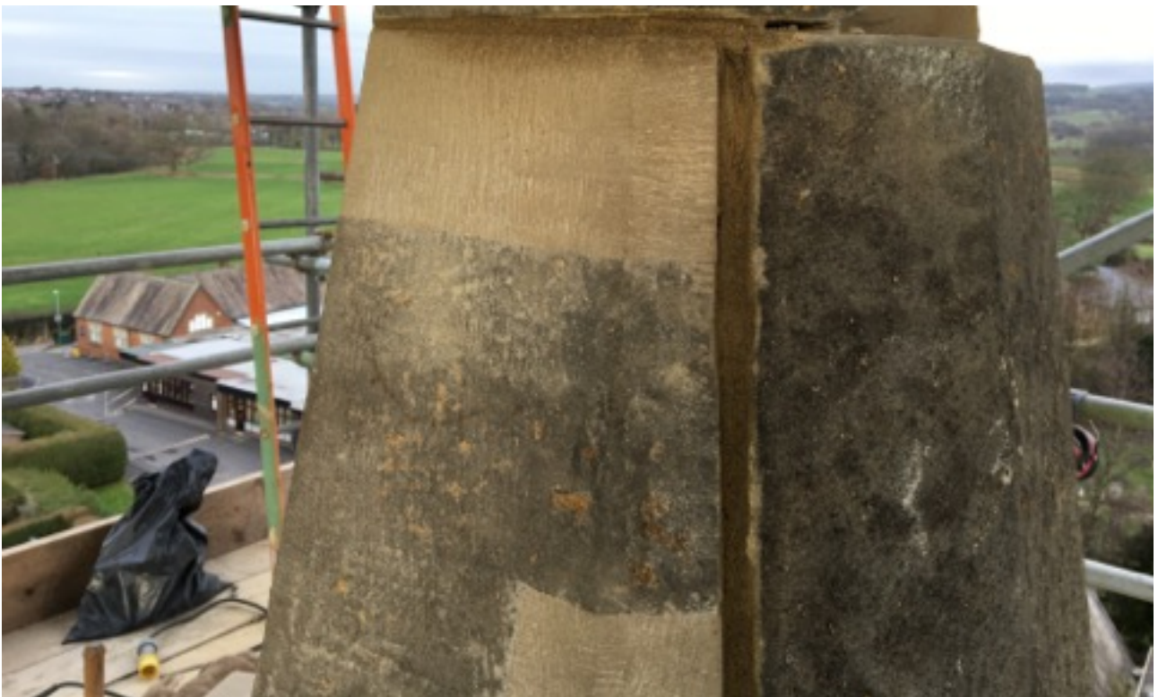
Pinnacle indented repairs
