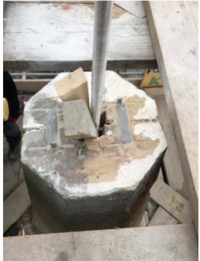
Pinnacle central 20mm rod and cramps between half stones
