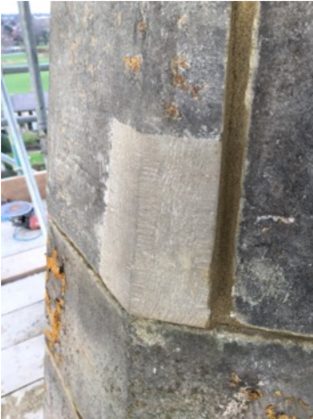
Pinnacle indented repair
