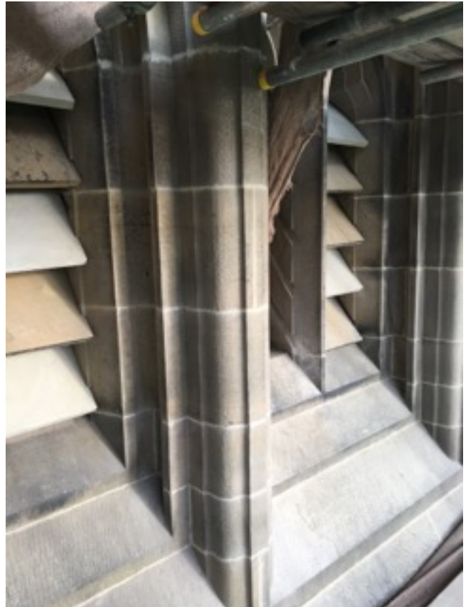
Belfry opening pointing and new louvres
