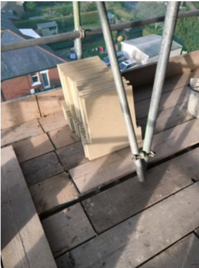
New belfry stone louvres
